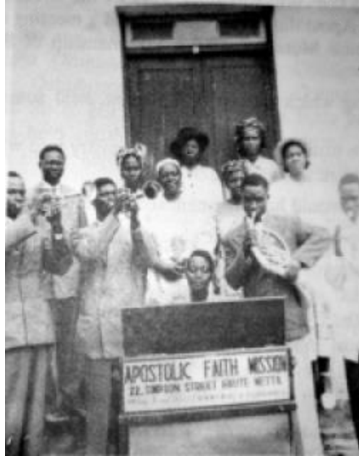
WORKERS IN FRONT OF 22 SIMPSON STREET
