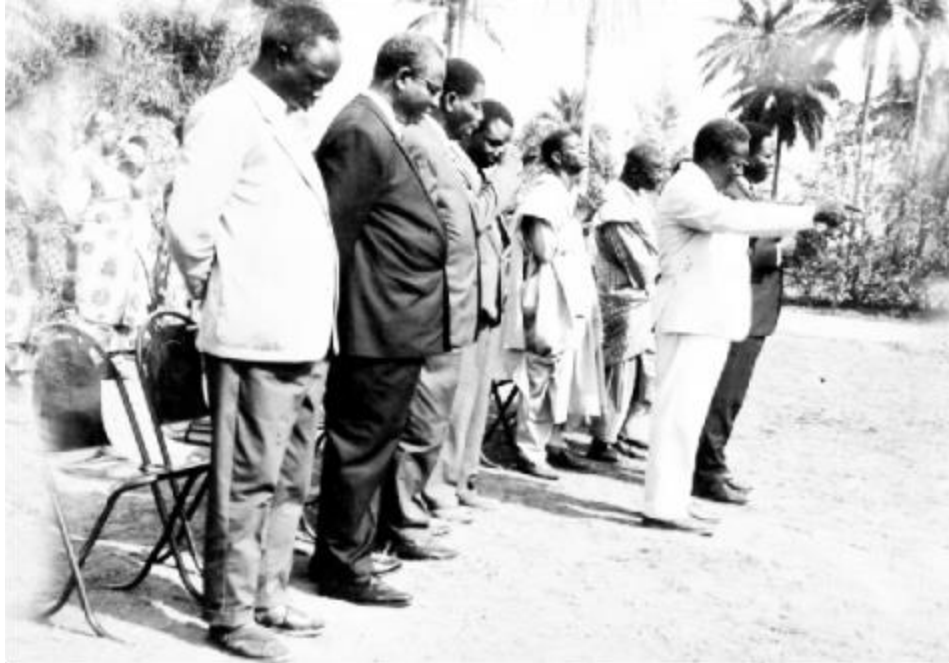
Foundation Laying Service of the Great Tabernacle Anthony Village, Lagos
