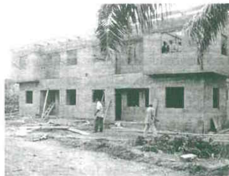
One of the residential quarters under construction
