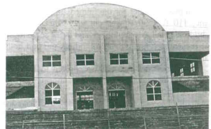
New Church Building under construction at Ilorin, Kwara/ Kogi District Headquarters
