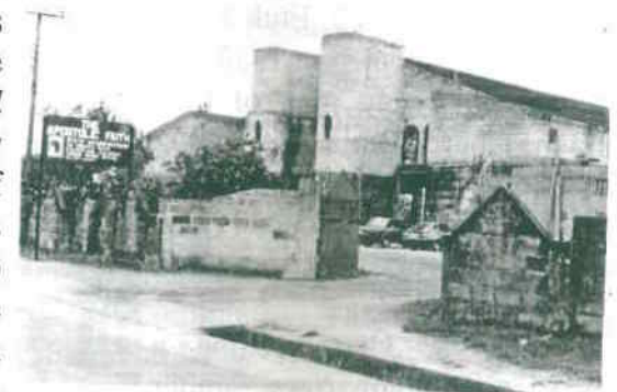
The Church in Calabar under construction
