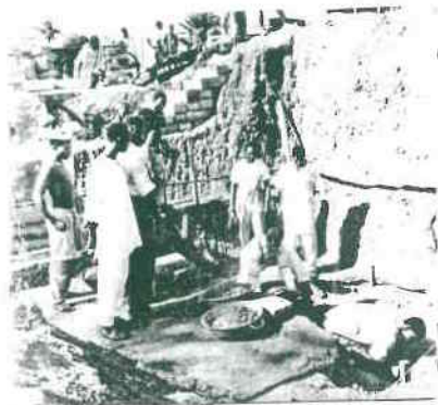
Digging of the Basement at 49, Moloney Street
