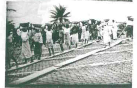
Construction work on the Great Tabernacle
