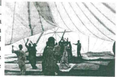
The tent church under construction
