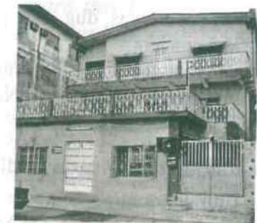
The New Building (Mission House) at 22, Simpson Street
