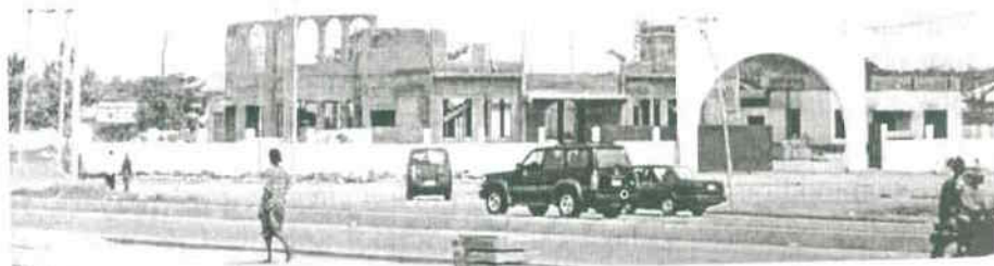
The New Church Building on Plot 456, under construction
