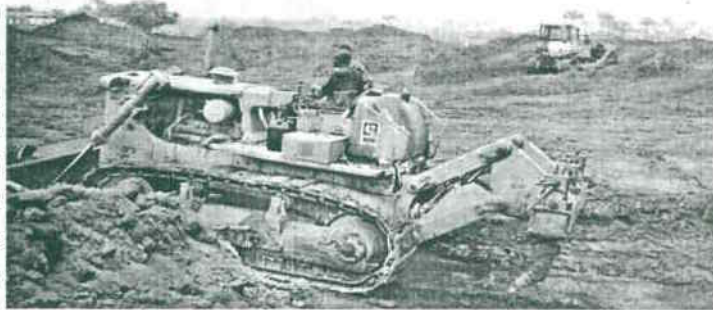
One of the bulldozers working on the site
